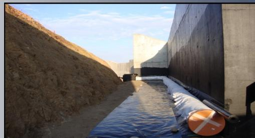
The membrane has a working temperature range of minus 20°C to plus 80°C. Terrethene can be welded with conventional hot air welding equipment or alternatively sealed with Terreseal double-sided Butyl tape.
